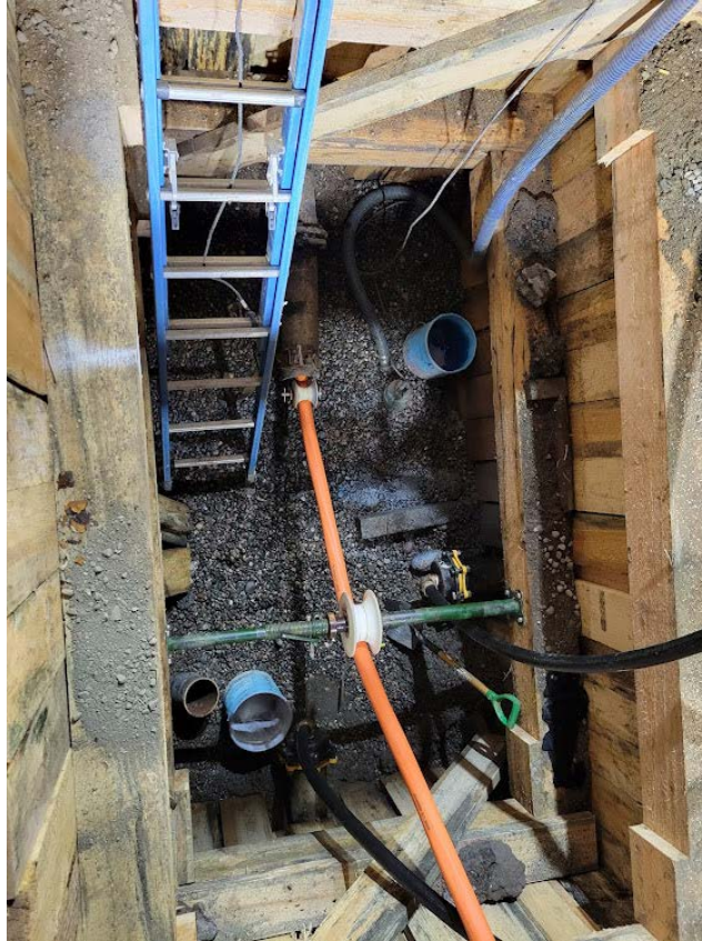
Figure 2.2: Lining umbilical with rollers.
